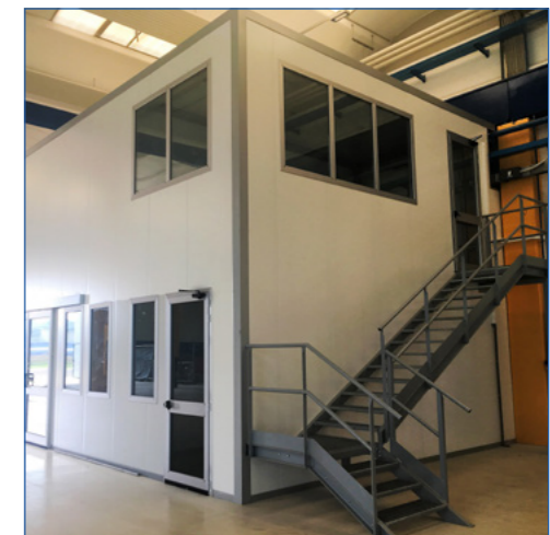
Laboratory and office on two levels
