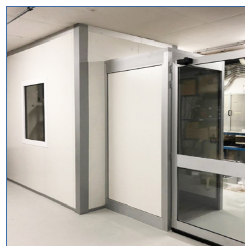
Entrances with double interlocked doors and cubicle compartments
